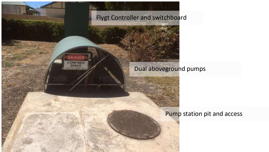
Figure 3 Penola aboveground pump station
