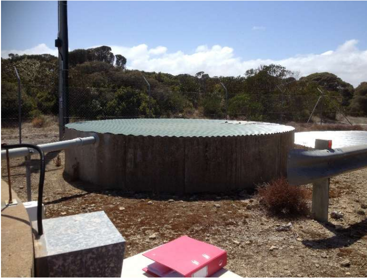
Figure 8 Sludge thickening tank at Southend WWTP
