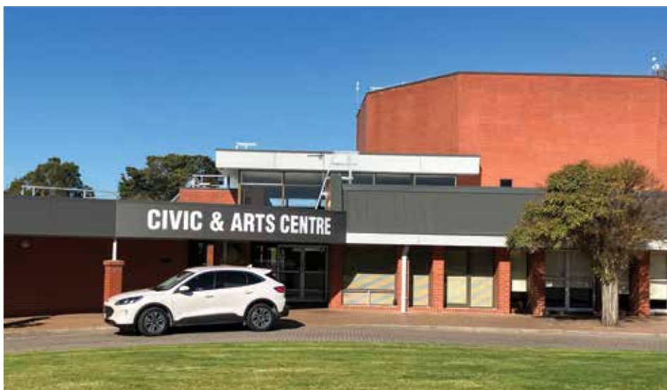
Millicent Civic & Arts Centre roof replacement.
