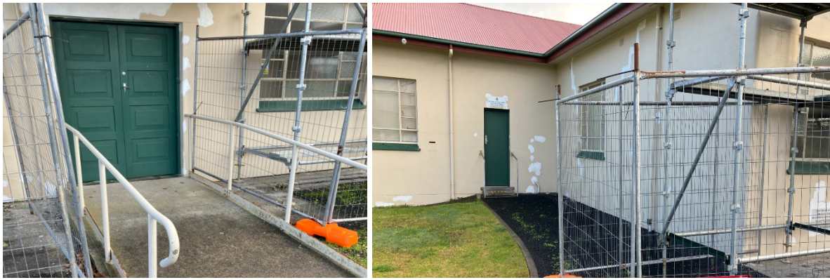
RSL Hall repairs
