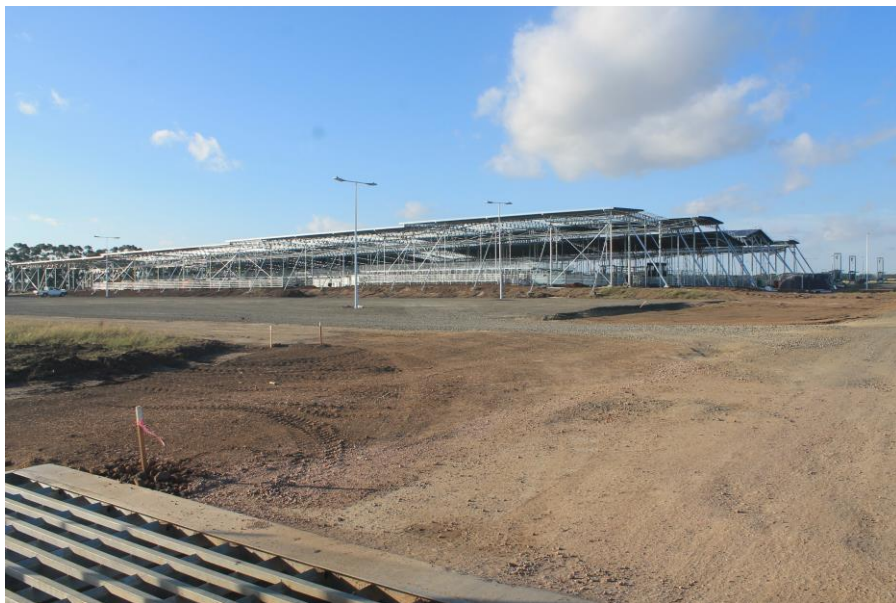
Figure 11 – View of Mortlake Saleyard under construction
