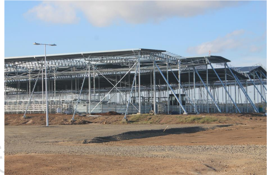
Figure 10 – View of Mortlake Saleyard under construction
