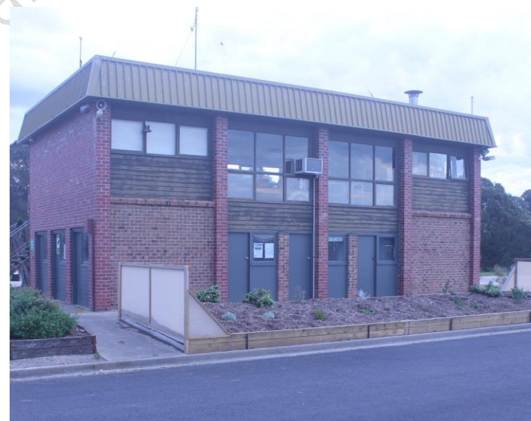
Figure 5 - Main office and amenities building
