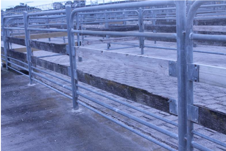
Figure 7 - Rails replaced as required
