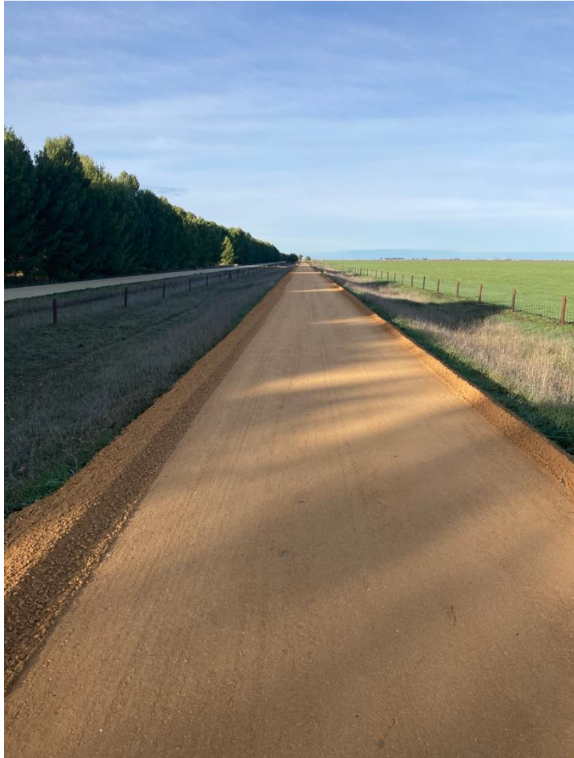
Coonawarra Rail Trail (stage 2) being prepared for sealing
