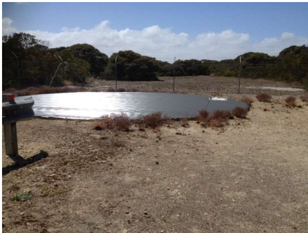
Figure 9 Decant tank at Southend WWTP
