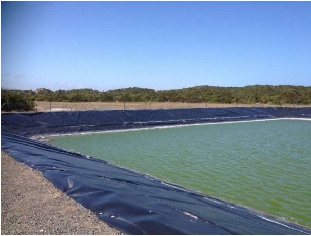
Figure 10 Storage lagoon at Southend WWTP and irrigation area in background
