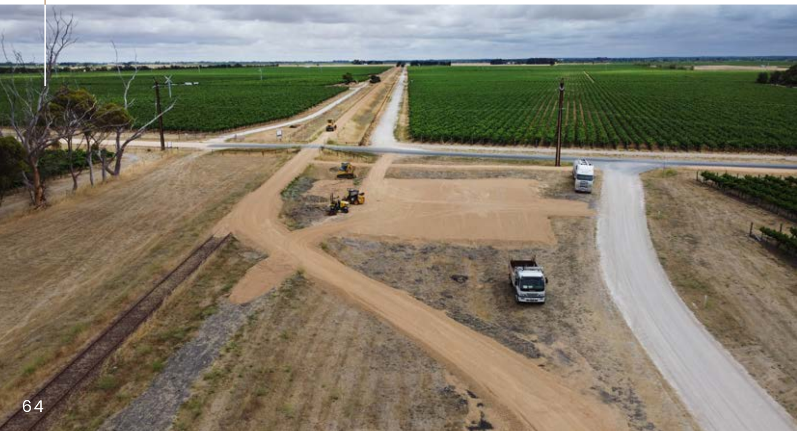
Preparing the Track - Coonawarra Rail Trail (Steve Chapple 2022).
