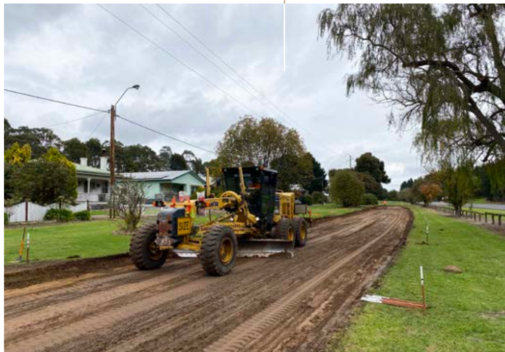
Mount Burr service roads upgrade.
