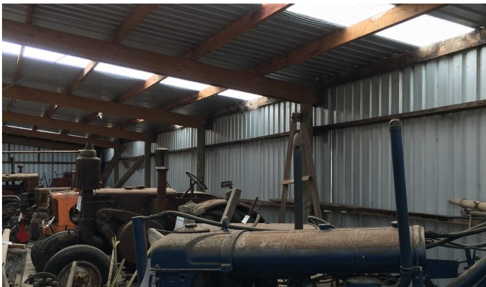
Machinery shed wall
