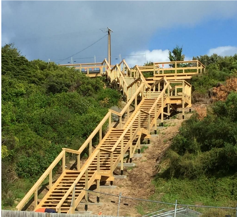
Wendy's Walk nearing completion
