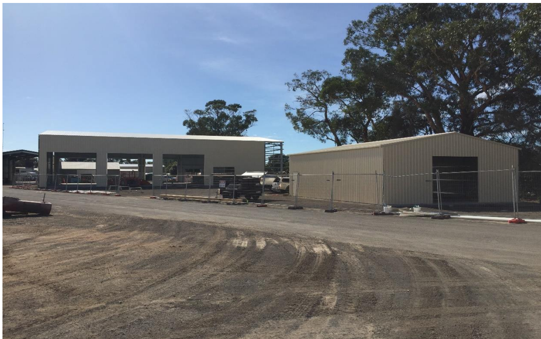
Millicent Depot Shed progress
