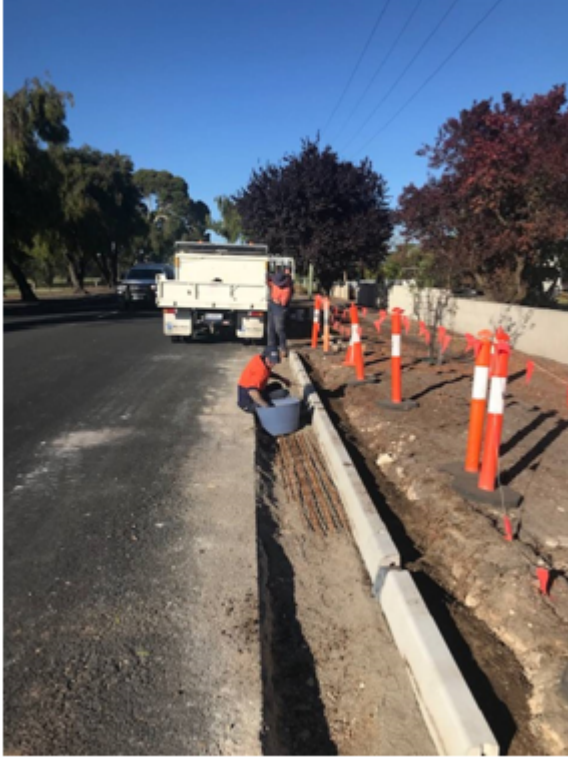
Ridge Terrace Kerb (in progress)
