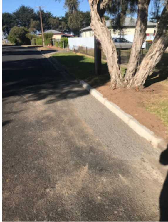
McCourt Street Kerb (completed)
