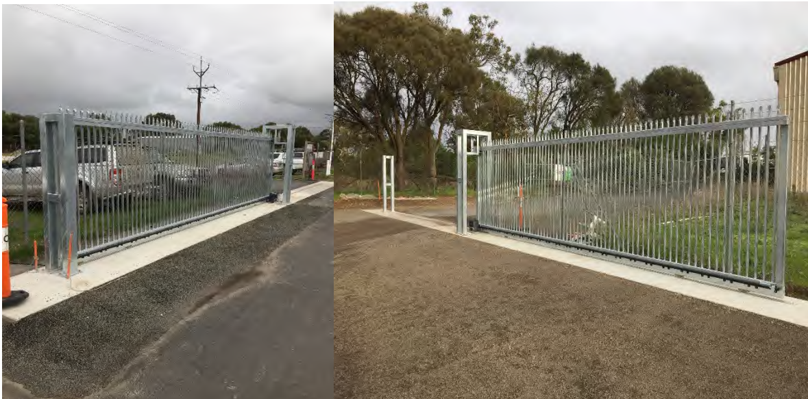
Depot access gates
