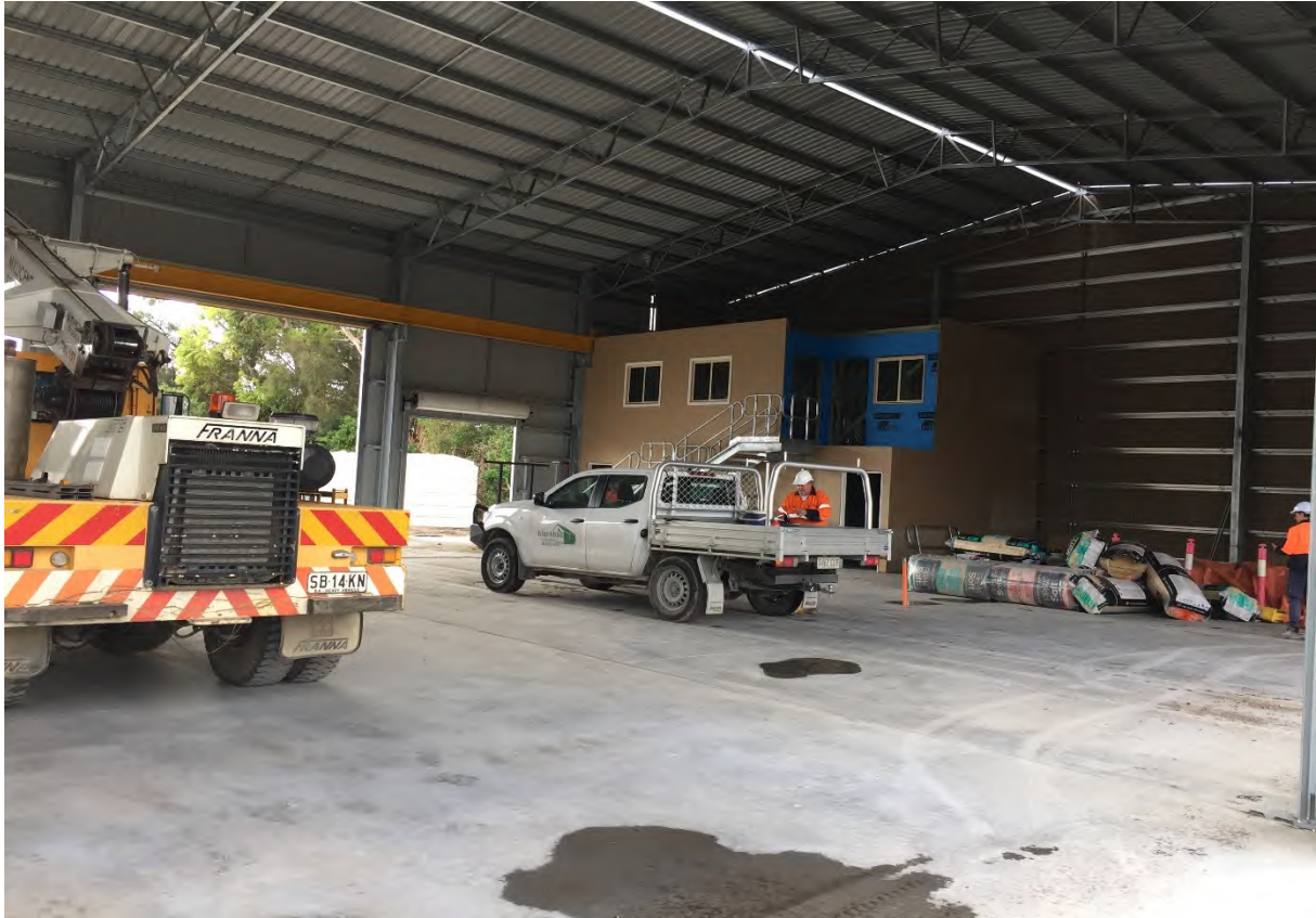
Millicent Depot shed internal fit out
