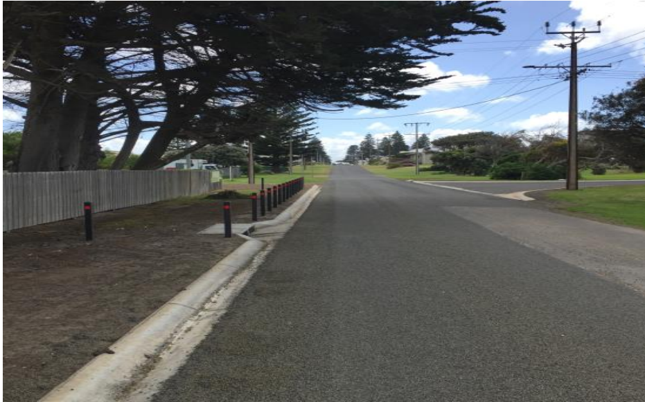
South Terrace upgrade
