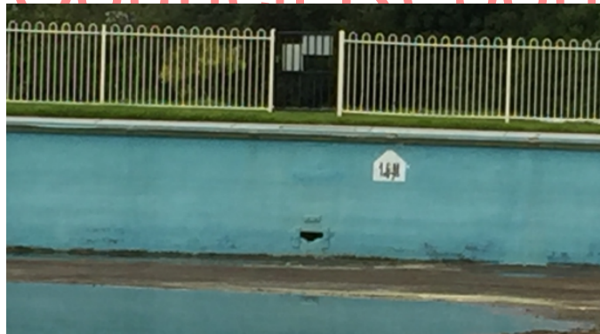
Current drainage outlet
