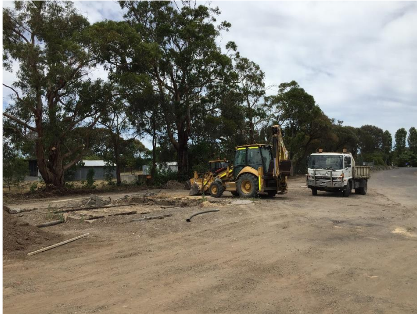
Millicent Depot Clean up and site preparation
