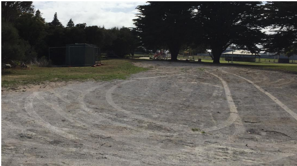
Civil work at centennial park
