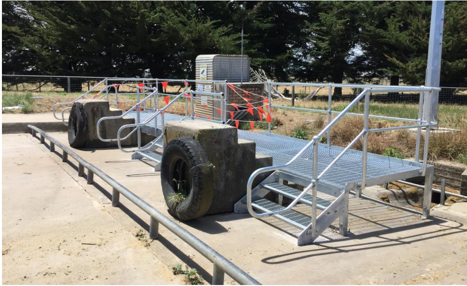
Truck wash upgrade
