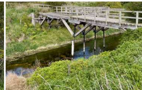
Narrow Neck Drainage Channel - Bridge is overgrown and unsafe
