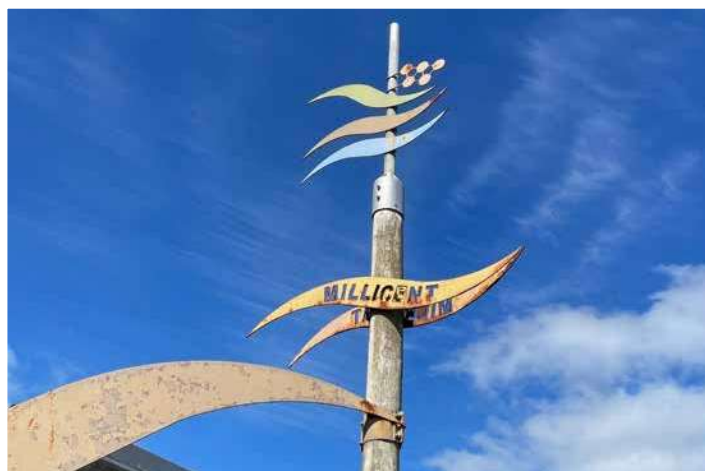
Millicent - 3 Panel Visitor Information Bay (Princes Hwy) - structure is in need of cleaning, rust treatment and painting
