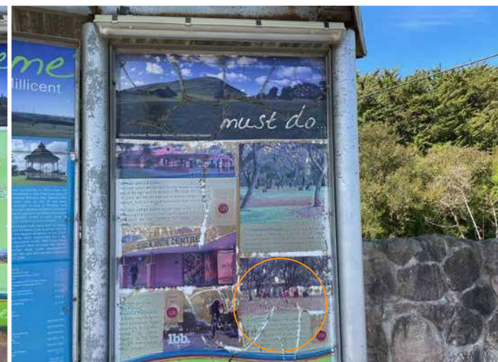
Millicent - 3 Panel Visitor Information Bay (Princes Hwy)- anti graffiti/UV laminate has wrinkled then broken down and failed
