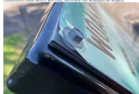
Woakwine Cutting - poorly installed interp panels (tech screws have lifted the interp panel vinyl, should have been blind riveted in place).
