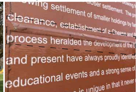
3) Glencoe Woolshed Visitor Information Bay - This results in the anti-graffiti laminate buckling and will eventually fail
