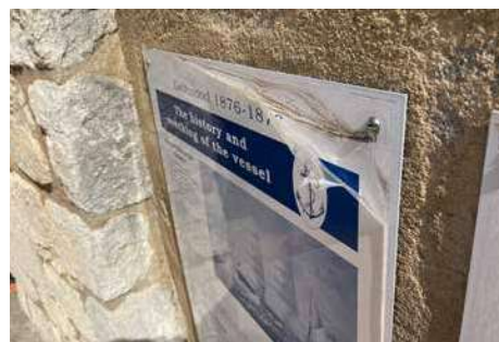
Gellwood Memorial - poorly fabricated sign panels (signs produced on colourbond steel which will rust, laminate not wrapped on edges)
