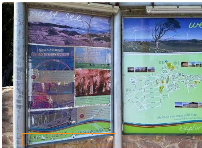
Millicent - 3 Panel Visitor Information Bay (Princes Hwy)- panel vinyl not wrapped and secured on edges and has shrunk and failed
