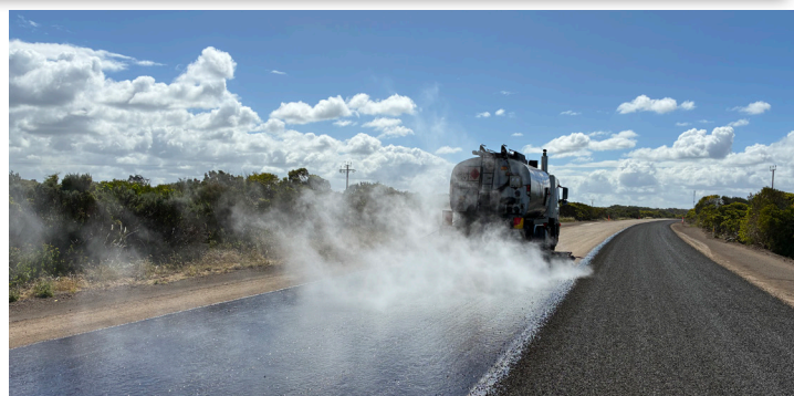
Southern Ports Highway reconstruction
