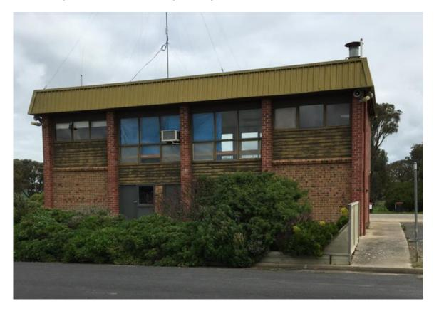
The building's condition is poor and requires either considerable investment to keep it watertight or demolition. Asbestos is present in the ceiling, in the floor tiles and wall sheeting and some parts of the kitchen. Southeast Asbestos has quoted to remove and dispose of the asbestos.
