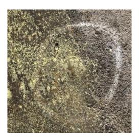
Towards the shallow end of the lake there are many areas that require reinstatement with evidence of cracking in the surface.
