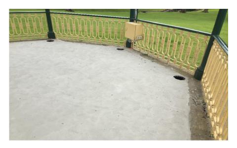
Rotunda new concrete inserts for lighting upgrade
