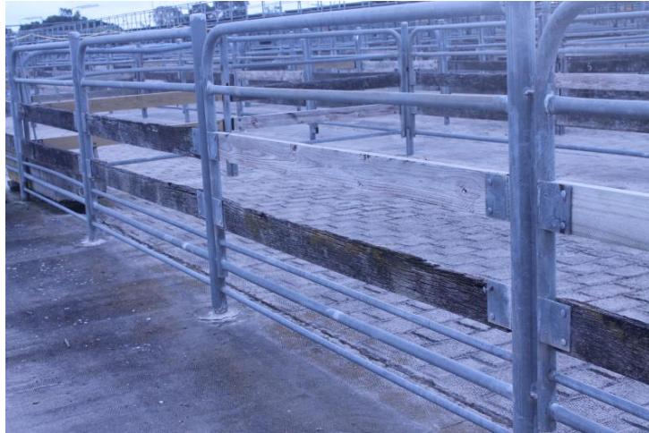
Figure 7 – Rails replaced as required
