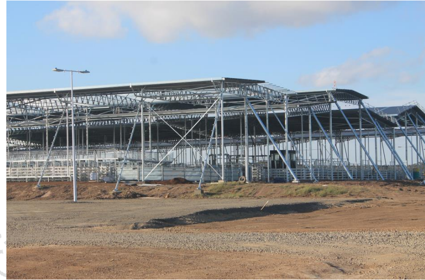
Figure 10 – View of Mortlake Saleyard under construction
