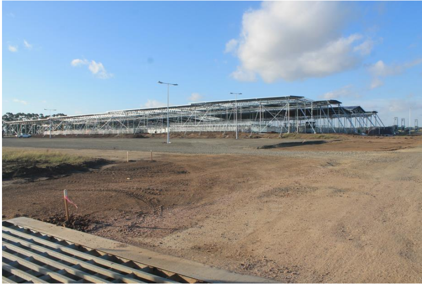
Figure 11 – View of Mortlake Sleyard under construction
