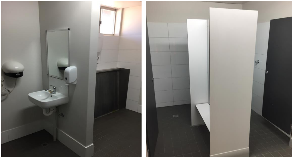
Stadium toilet upgrade
