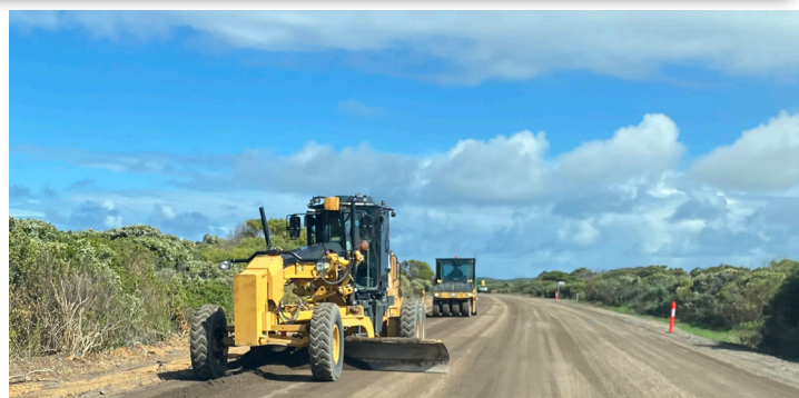
Southern Ports Highway reconstruction
