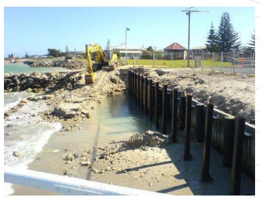
Photograph 3.3 – View to the South (from the Jetty) of the vertical seawall construction. (Source: Author, November 2006)
