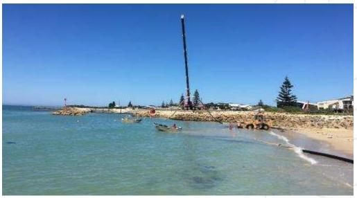
Photograph 5.12 – Relocation of the dredge discharge pipe using the crane and a front end loader on the beach (Source: Author, March 2017)
