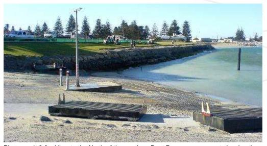
Photograph 3.9 – View to the North of the previous Boat Ramp arrangement showing the relatively steep armoured revetment wall. (Source: Author, November 2006)
