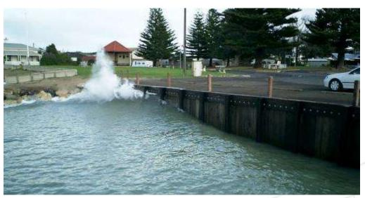
Photograph 3.4 – View of a reflected wave forming at the timber seawall adjacent to the jetty during large swell conditions, Beach 8 (Source: Author, May 2007)
