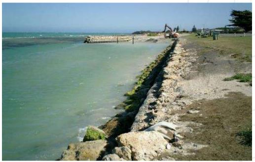
Photograph 3.8 – View to the South of the previous Boat Ramp arrangement showing initial gabion basket revetment wall with additional rock protection. (Source: Author, November 2006)
