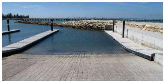
Photograph 5.1 – Boat ramp and concrete retaining wall. The additional set of floating pontoons creates a 4<sup>th</sup> lane for vehicle access. (Source: Author, March 2017)
