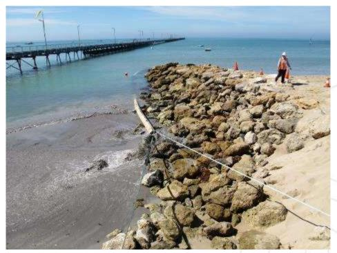
Photograph 5.10 – Sand slurry discharged onto the jetty beach with the HDPE pipe tethered to the vertical seawall using a bridle arrangement (Source: Author, March 2017)
