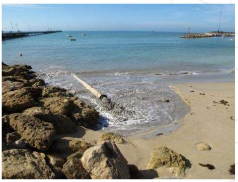
Photograph 5.9 – Dredge pipe placing sand slurry on the lower beach. The beach was almost immediately restored after pumping was ceased in this location (Source: Author, March 2017)
