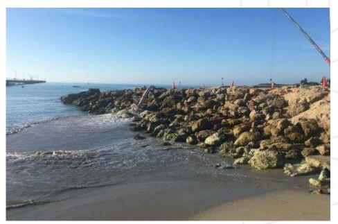
Photograph 5.7 – Sand slurry pumped onto the rock groyne adjacent to the jetty beach, with the build-up of sand evident along the length of the groyne (Source: Author, March 2017)
