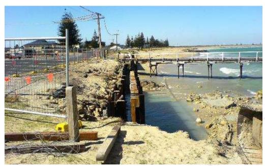
Photograph 3.2 – View to the North of the renewal / replacement of the vertical seawall adjacent to the jetty. (Source: Author, November 2006)
