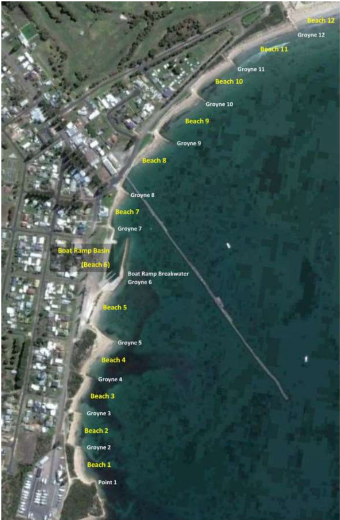
Figure 1: Numbering of beaches and groynes
